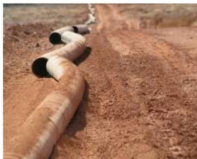
Once the pipe was installed, the Dalkeith team then cut and joined it into the main bore line using isolation valves to stop the flow. At the same time complete a road crossing without disruption the ore trucks dumping material. It was a co-ordinated process that required no mistakes from the civil operators to the welders completing the pipe works.
